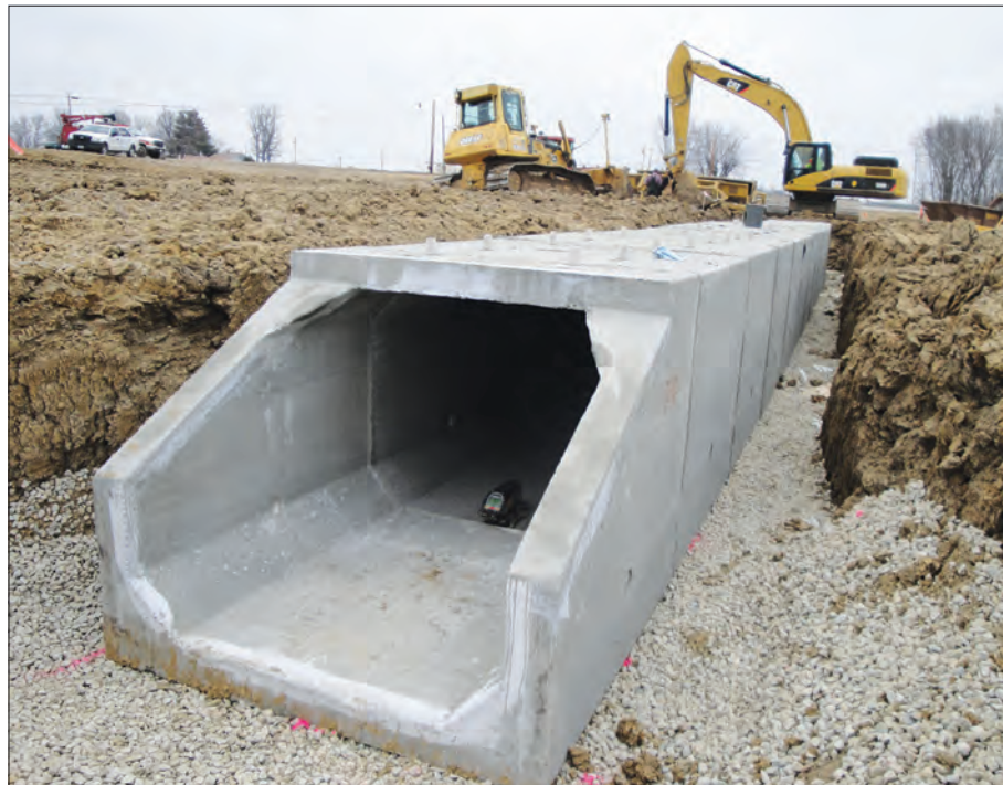
Box culvert drainage project by Quigg Engineering.
