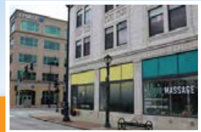
The historic Kerasotes building at Sixth and Washington got two new tenants as Moxie Massage expanded in both in square footage and its services and Physiotherapy Professionals opened a second location.
