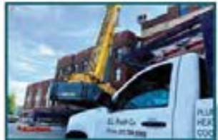
Blessing Hospital (Quincy)
