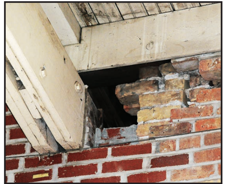
Bricks are missing from key structural points inside the Coliseum.
