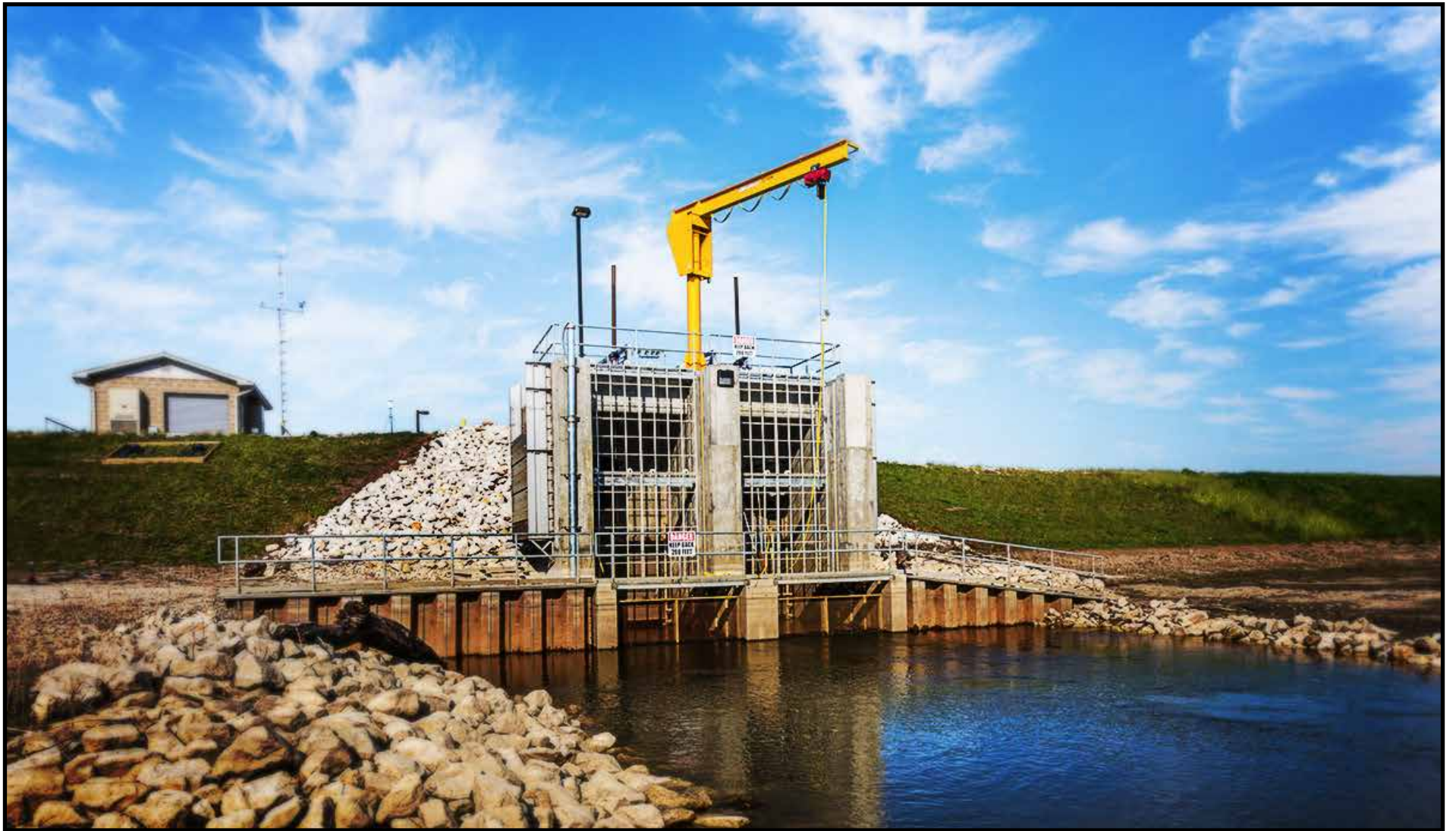
The water control structure, with its sluice gates, now allows the Emiquon, a 5,500-acre wetland area, to be reconnected to the Illinois River, providing environmental benefits to both the river and the wetland.
