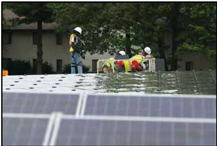
Workers install solar panels on a carport at Crawford, Murphy & Tilly, Inc. in Springfield. In the foreground are some of the many solar panels on the company's main building.
