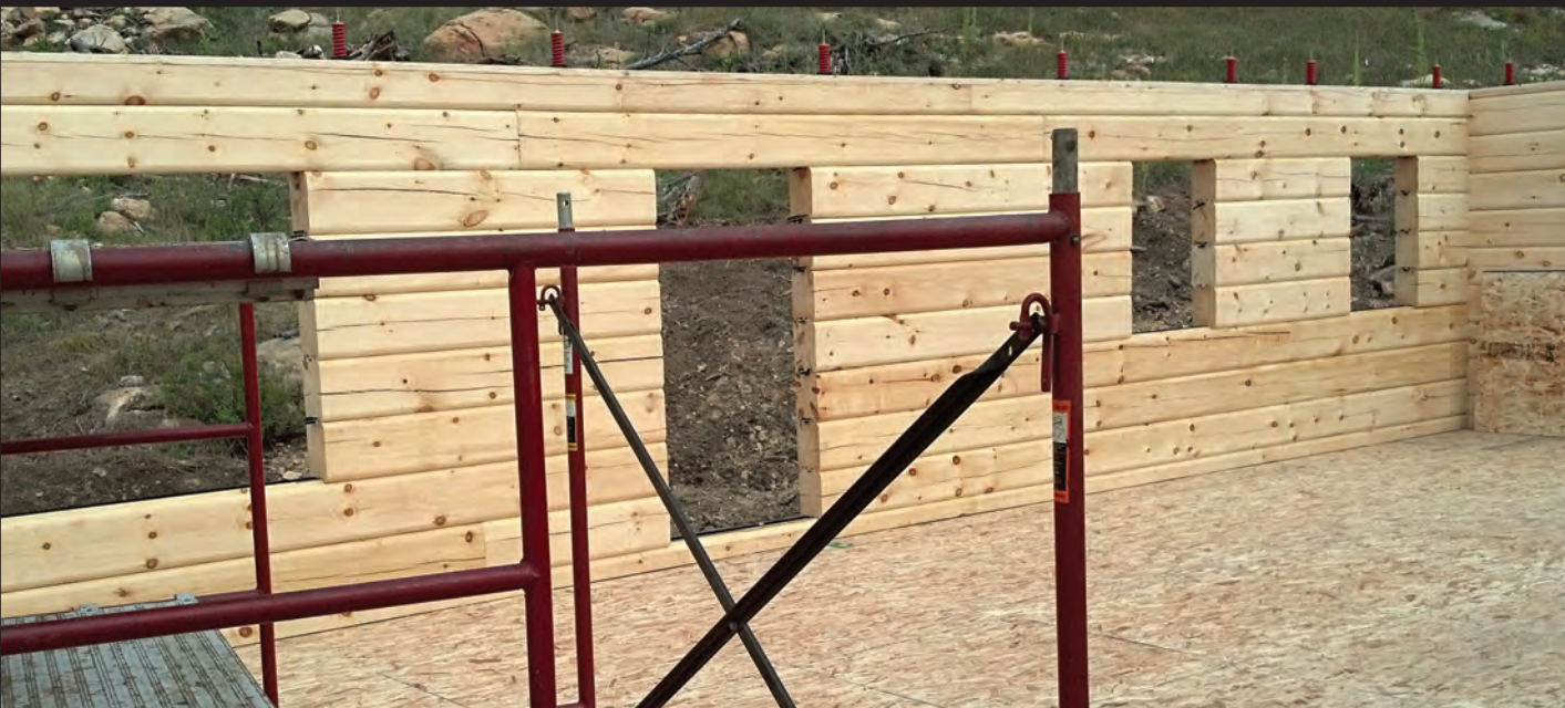
A vacation rental going up near Rapid City, South Dakota. The logs are the 8" x 12" pre-primed, rounded groove design ready for a customer applied True North finish.
