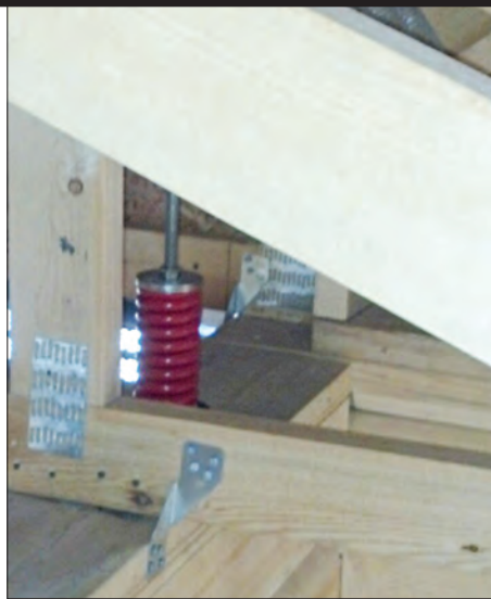
The red spring is the top of one of the many True North Log Homes "Log Lock Compression Systems" installed in the exterior log walls. Applying 2500 pounds of downward pressure, this log lock system is why True North can give a 25-year "ZERO" air infiltration warranty.
