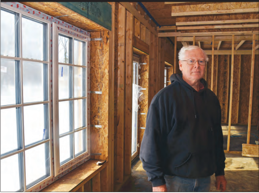
David Cation is building a "passive home" in Chatham
