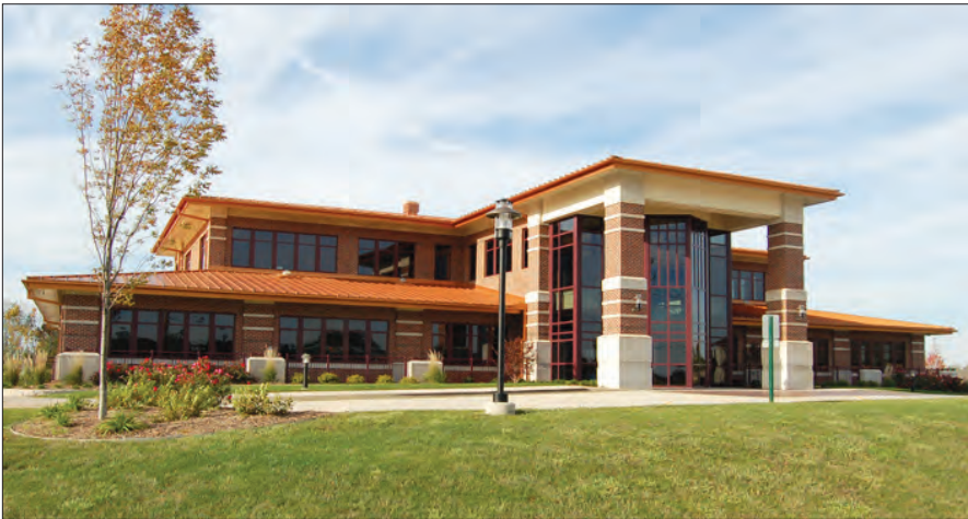
Allen Henderson and Associates, Inc. provided the complete structural designs for the new headquarters of the Illinois Municipal Electric Agency. The core of the building is designed to resist forces produced by an F-5 tornado, ensuring the agency can remain operational if such an event were to occur.
